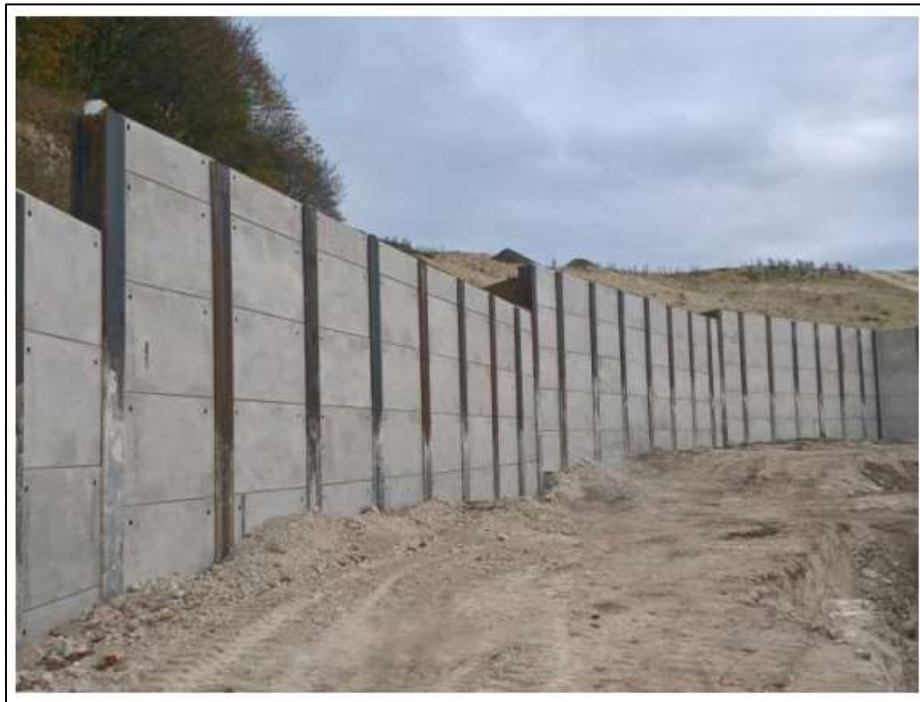
Insert 3: King Post Retaining wall example
